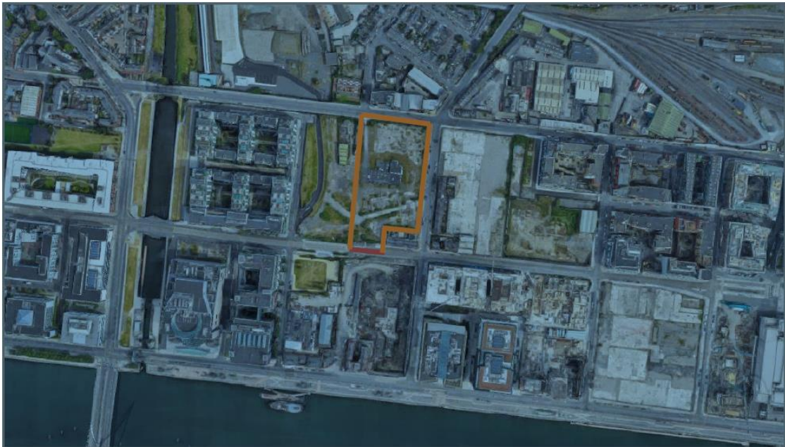
Figure 1.1 Site Location (Grid Reference O 176 346)
